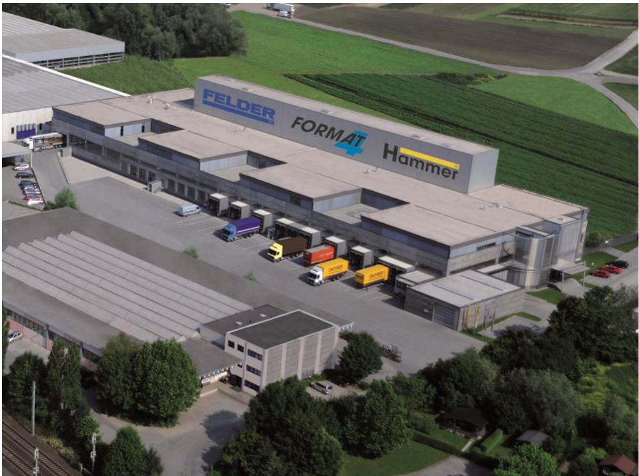
Felder Group factory and head office in Hall in Tirol
